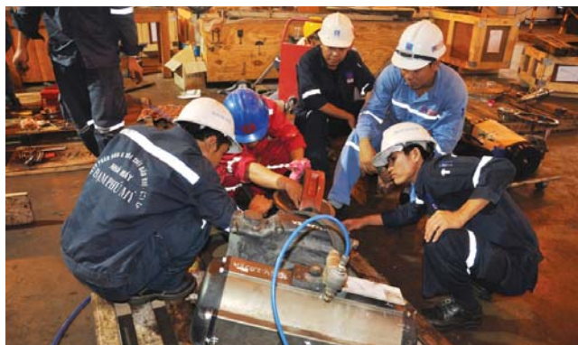
The overall maintenance was carried out at Phu My Fertiliser Plant. Photo: PVFCCo
